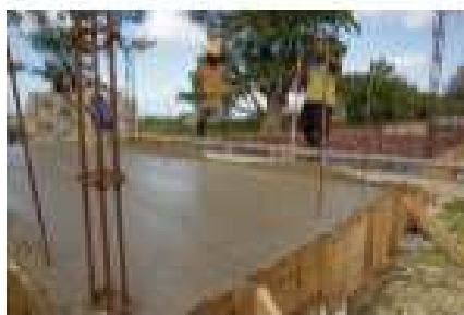
The first portion being smoothed
