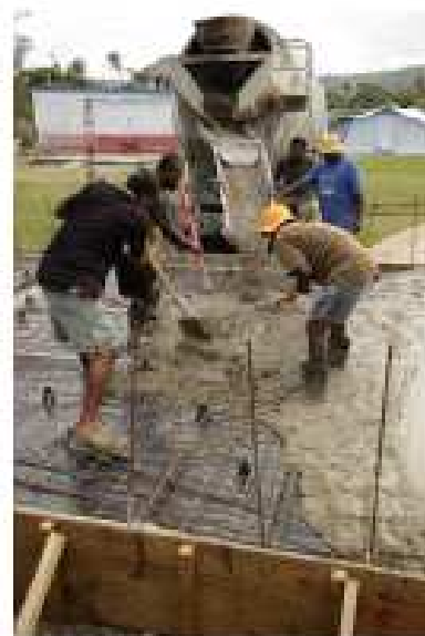
Concrete poured for the base slab
